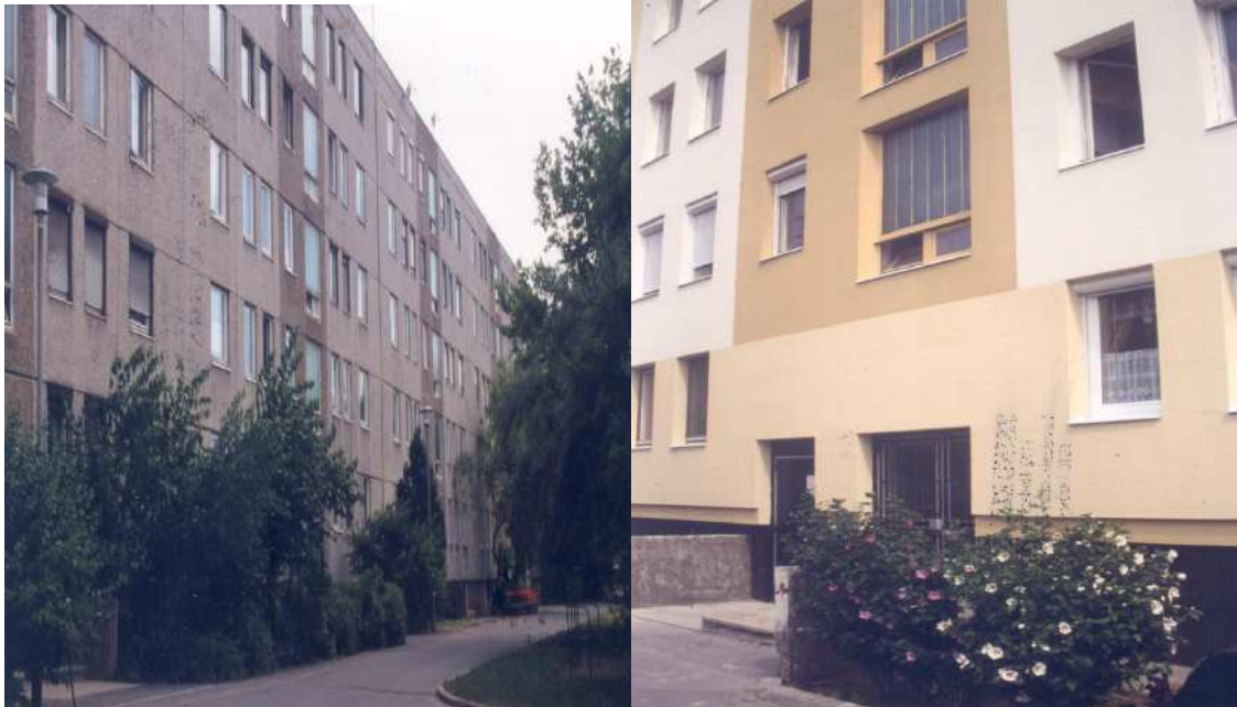
Illustration 2 The “Csombor utca” building before and after retrofit
