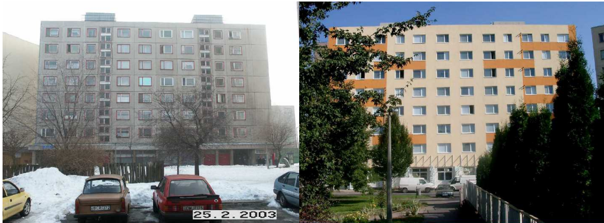
Illustration 1 The “SOLANOVA” panel building before (left) and after (right) renovation
