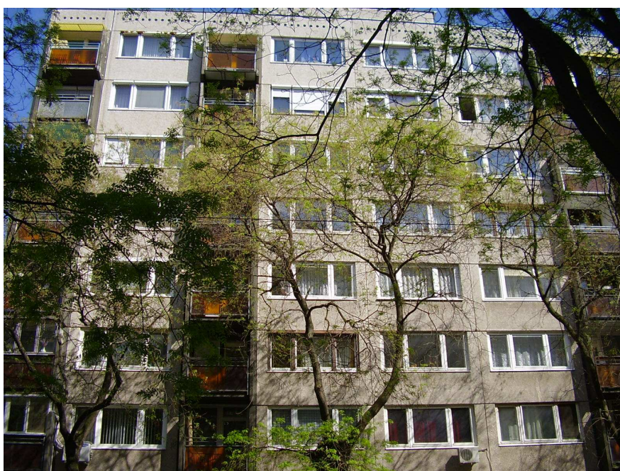
Illustration 5 A building constructed using industrialized technology (Budapest, Hungary)
